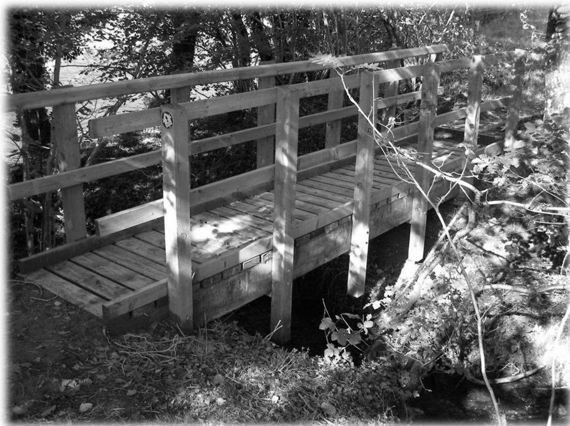
Timber Footbridge, Llanfair ar y Bryn
